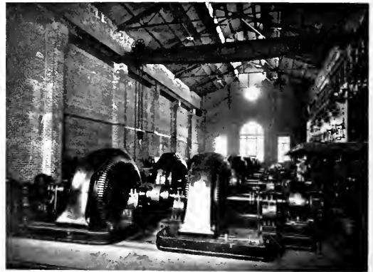
FIG. 2.—FIVE FREQUENCY CHANGERS AT MONTREAL.
